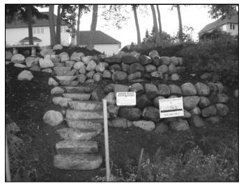
Water run off is captured in a series of rain gardens where water is filtered before it enters the lake.
