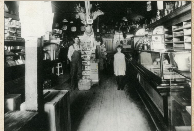
Interior of Miller Store
